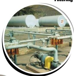
In bulk applications, oil can easily get contaminated with built-in, ingressed or induced particulate and bacteria growth. Filtering oil in bulk storage tanks and reservoirs makes it easier to keep it clean in machines and hydraulic circuits.
